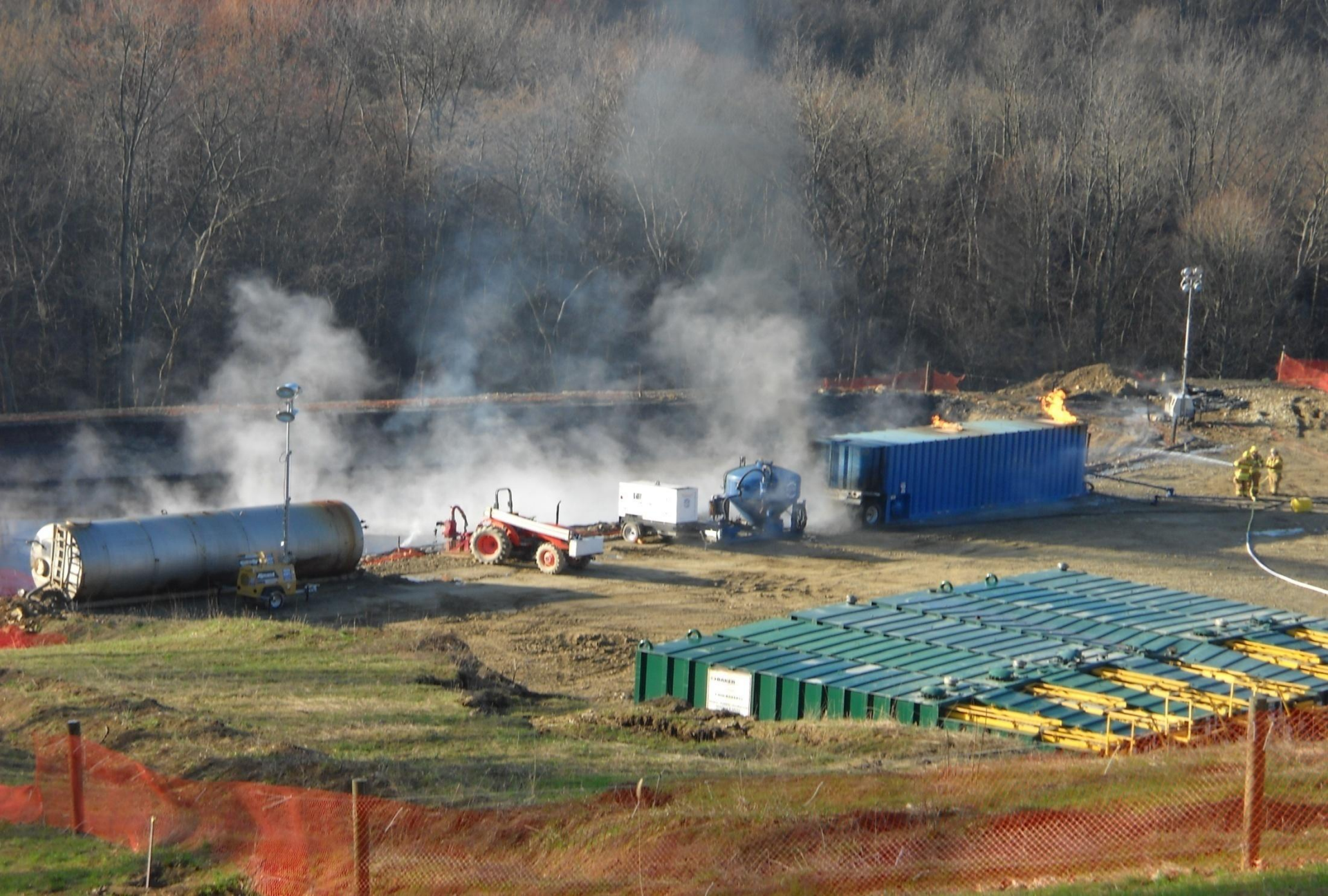
Fracking Pond Fire – Hopewell Township, PA – reported by Post Gazette April 1, 2010
